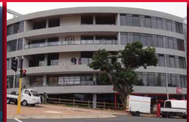
Front of the building. Pedestrian entrance is to the right of Vida.
